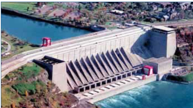
Hydroelectric plant on the Niagara River
